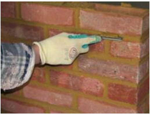
pointing the joints in the brickwork using an iron is one way to point brickwork
