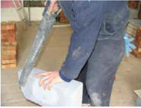
using a block saw for blocks
