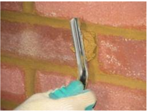
pointing the joints in the brickwork using an iron is one way to point brickwork
